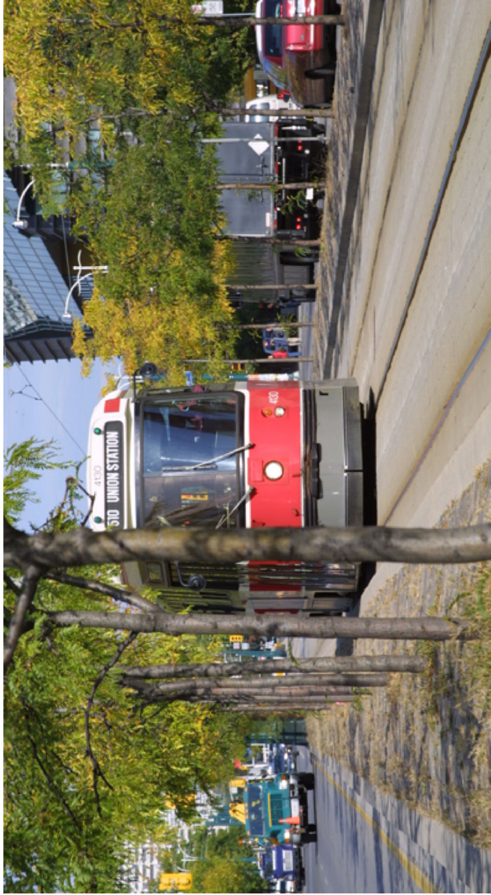
Exhibit 6 Example of Streetcar Right-of-Way Protected by Landscape Median (Spadina Avenue)
