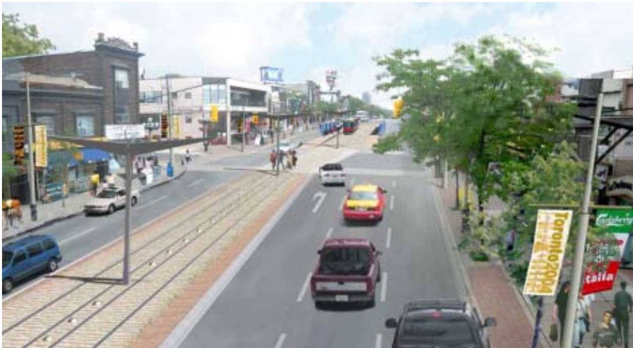
Figure 22: Perspective View of Preferred Alternative, featuring raised trackbed with rolled curb, center pole and transit shelter.
