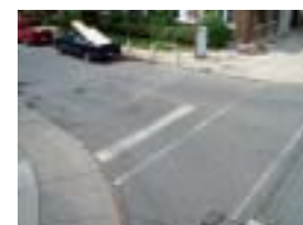
43. Poorly defined crosswalk
