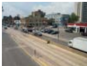
10. Bathurst Street intersection
